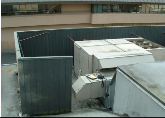
Field conditions must be verified
