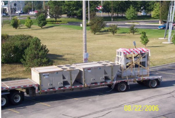
Equipment arriving on site
