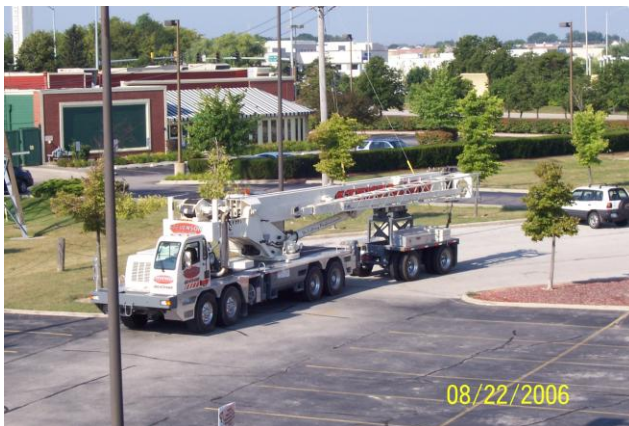
Crane arrival at the jobsite
