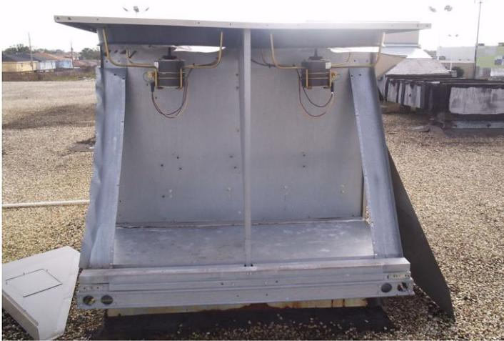
*This relatively new unit was stripped by vandals for the scrap value of the copper coils. An excellent example of a reactive replacement candidate.*
