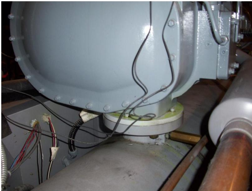
Refrigerant leak discovered on cooling inspection. This will take 2 days to repair. Can you afford the down-time during the cooling season?
