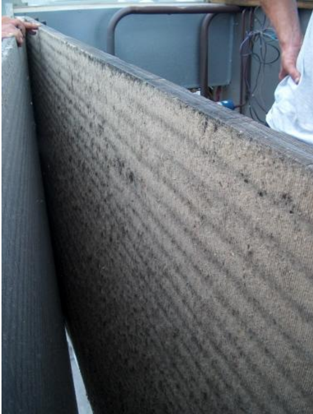
Dirty Condenser Coil Increases Energy Usage
